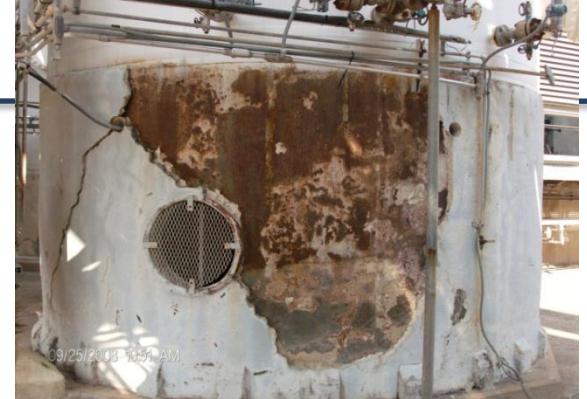
CUF: Corrosion under fire proofing
